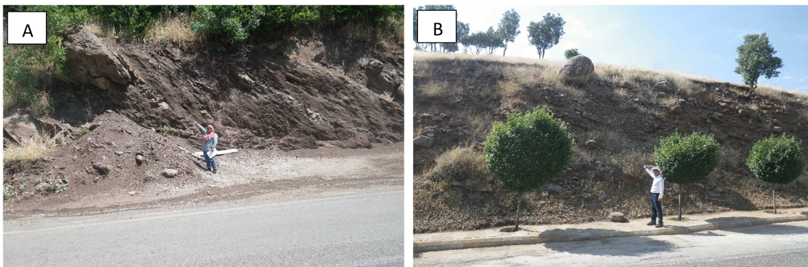
Figure 13: a, shows the crushed rock mass at site No.15 b, quaternary deposit at site No.2
