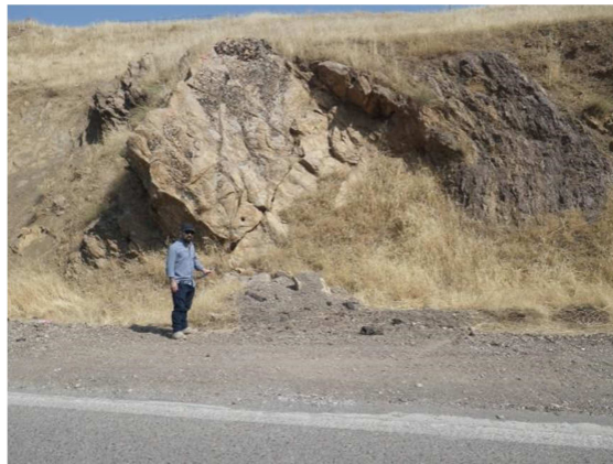
Figure 8: front view of site No.4 shows moderate (LPI) hazard category
